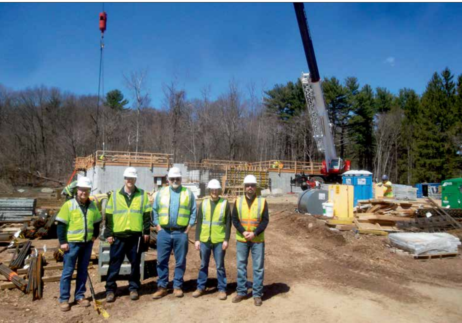
Construction team leaders, from left: RH White Project Manager Jamey Pedro; AECOM Project Manager Jim Mitchell, Construction Manager Steve Small, and Project Engineer Tom Herer; and Connecticut Water Company Construction Manager Nick Meder.
